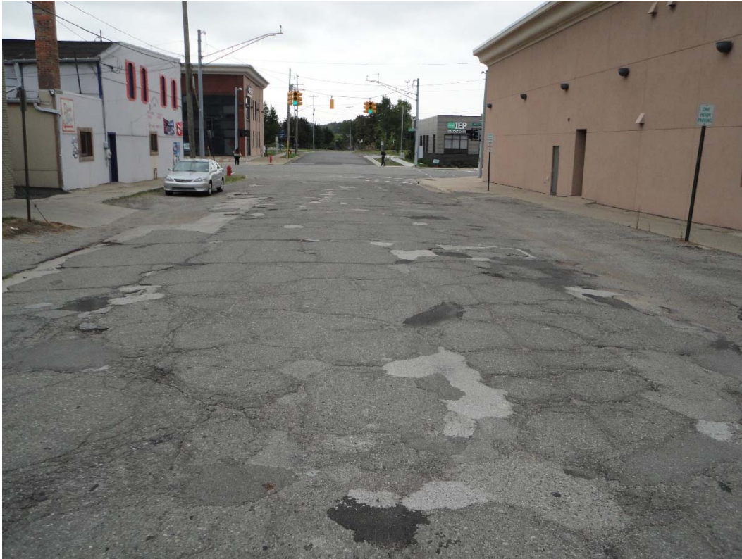
Photo 1: Perrine Midblock of Michigan to Pearl looking south to Michigan Ave
