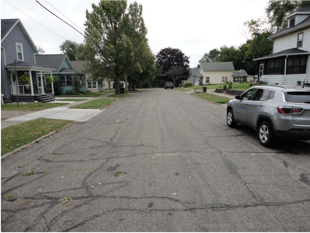
Photo 2: Arnold, in front of 119 Arnold looking east toward East End
