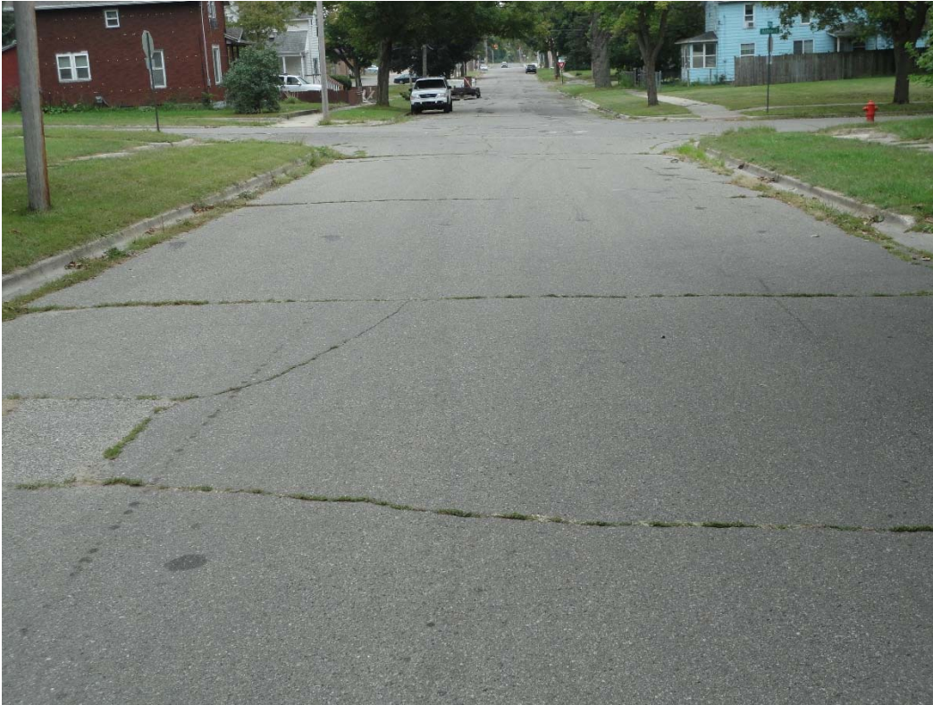
Photo 5: Perrine Midblock of Homewild to Burr looking south at Homewild St
