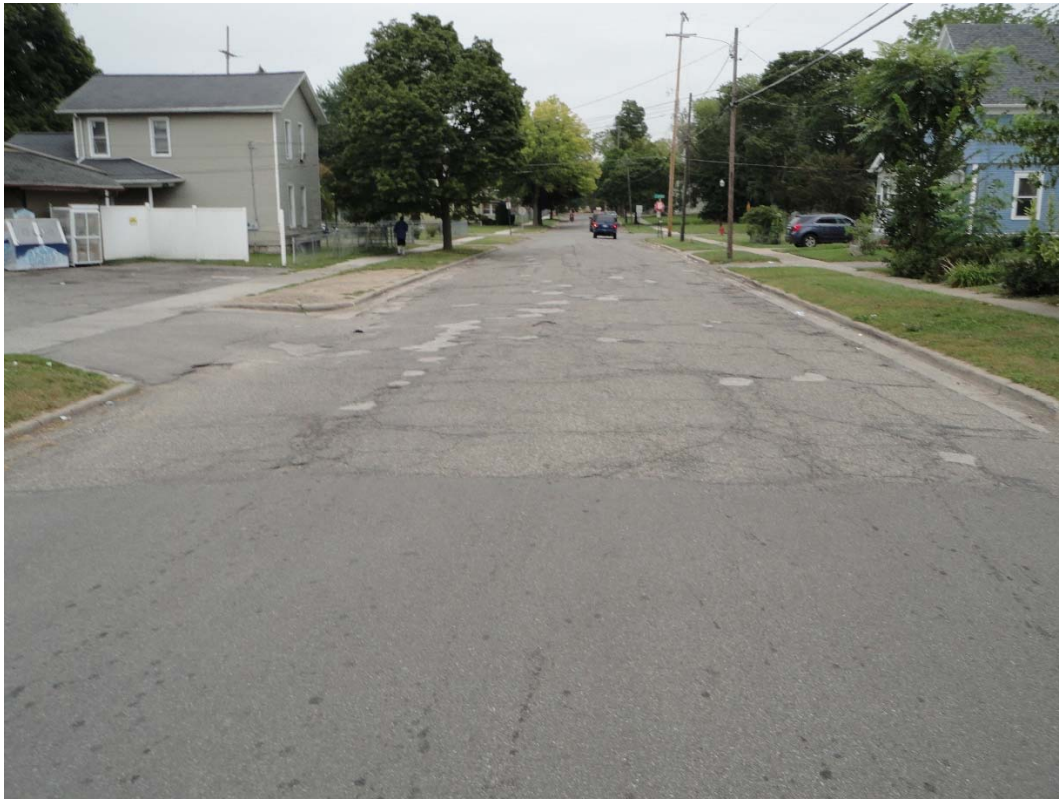
Photo 1: Biddle Street at Greenwood looking east toward Jackson Street
