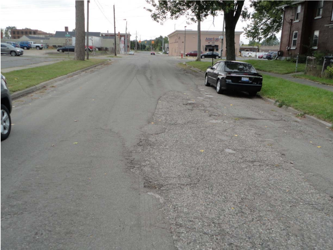
Photo 1: Perrine Midblock of Pearl to Detroit looking south at Pearl St
