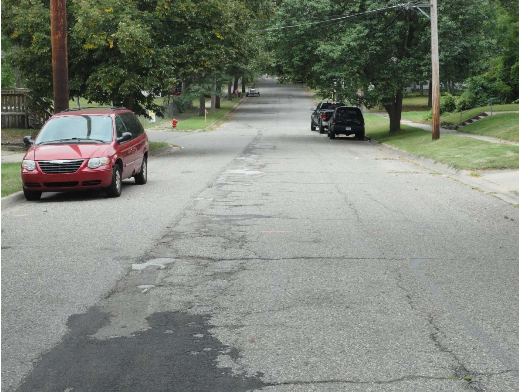
Photo 7: Burr Midblock of Perrine to State looking west to Perrine
