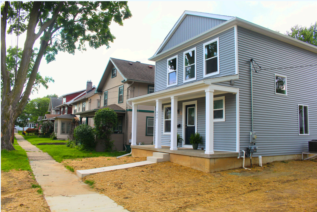
Second home completed through the 100 Homes Program on McBride Street in July 2024.
