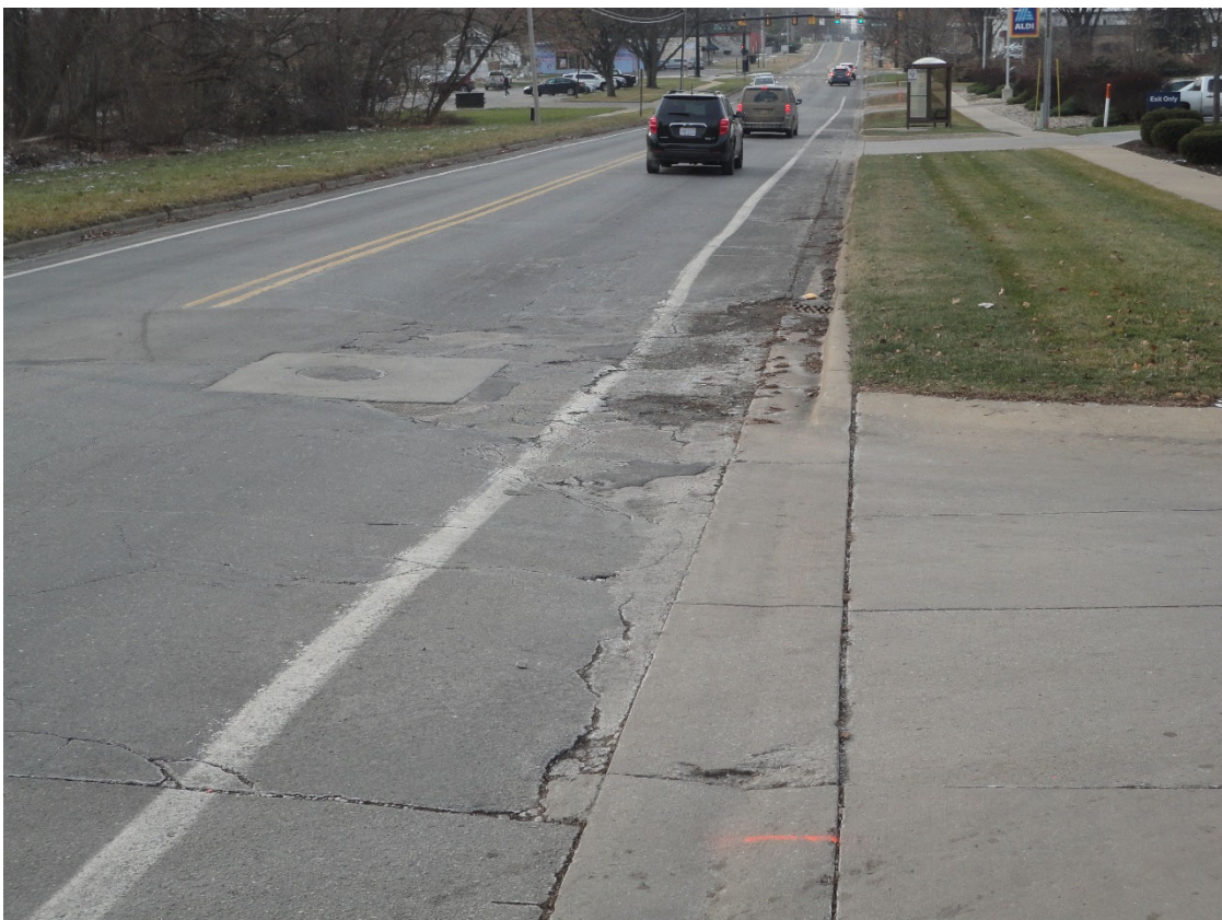
Photo 4: North St looking west from Hibbard St at north curb line
