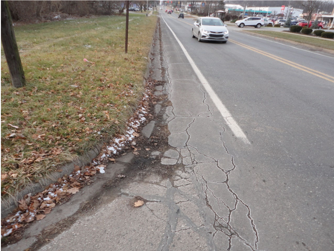
Photo 5: North St looking west from Hibbard St at south curb line
