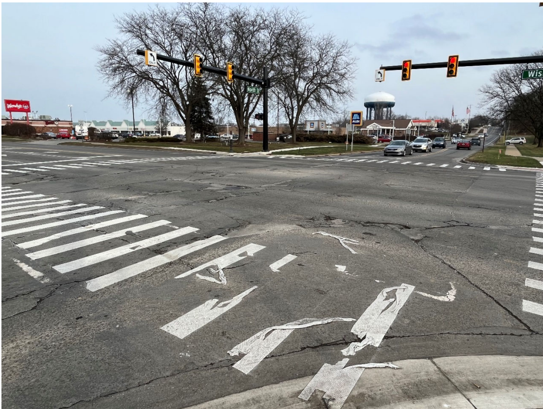
Photo 8: North St and Wisner St intersection looking northeast
