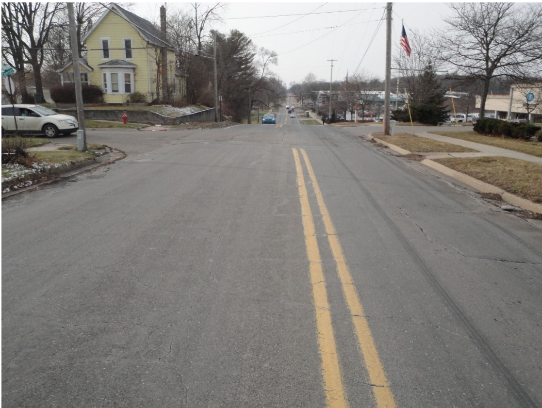
Photo 2: North St looking west toward Center St
