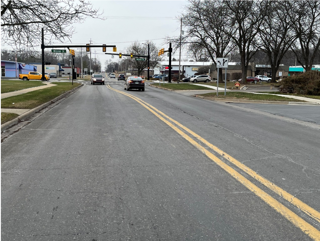
Photo 7: North St looking west from bank drive
