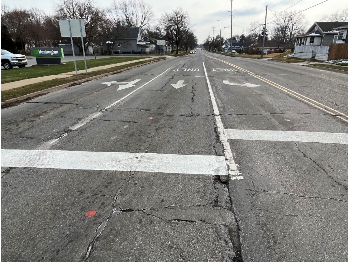
Photo 9: Wisner St looking south from North St
