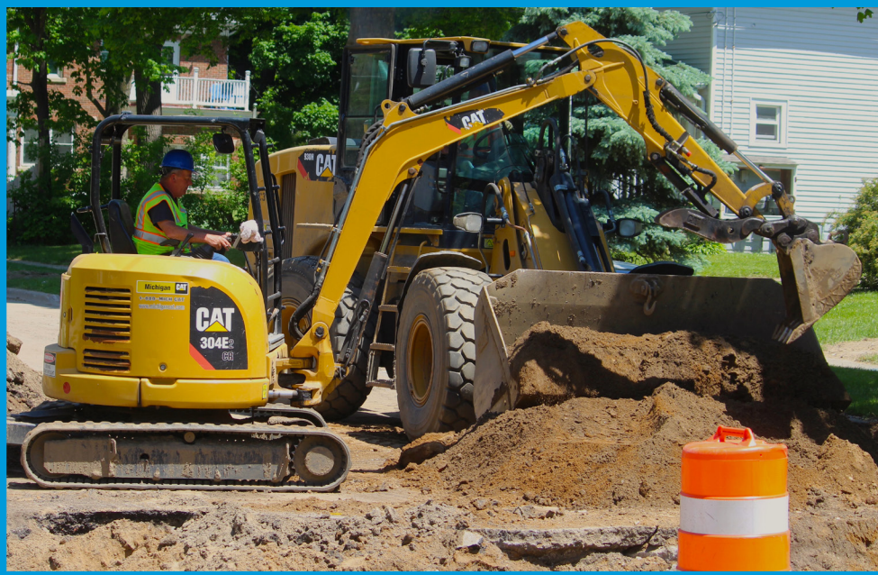
Water main and lead service line replacement project on S. West Ave.
