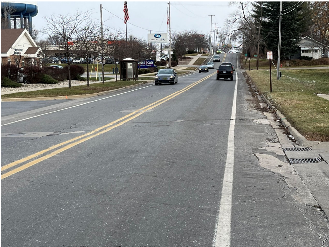
Photo 6: North St looking east from bank drive
