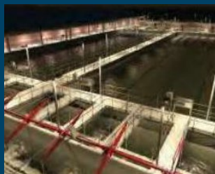
Huntsville, AL Surface Water Treatment Facility (24 MGD, $90M)
