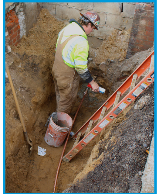
Lead line replacement on E. Michigan Ave.
