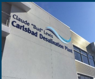
Carlsbad, CA Seawater Desalination Program (50 MGD, $900M)
