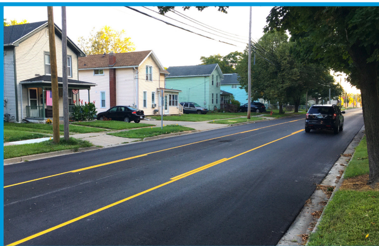
New pavement on Greenwood Avenue.
