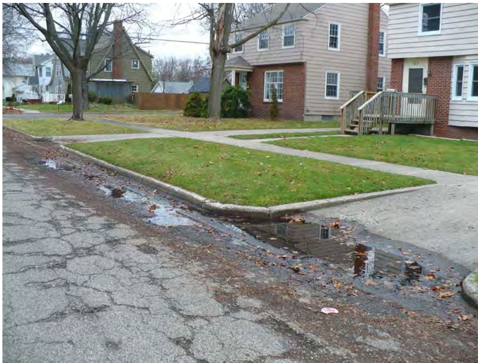
Photo 4: East curb south of Elmwood
