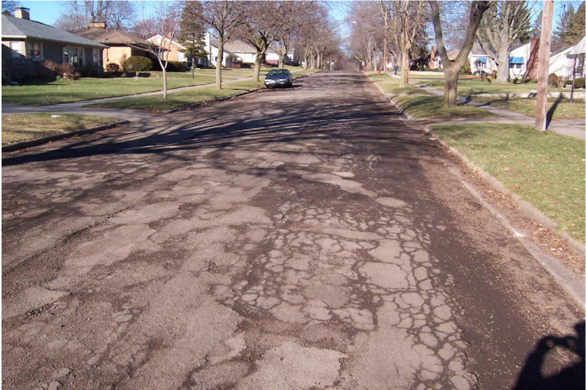
Photo 5: Facing north on Durand near Elmwood
