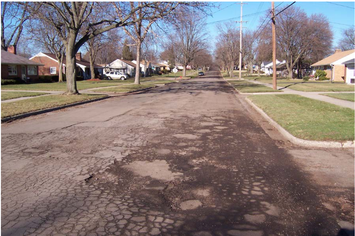
Photo 4: Facing north on Durand mid-way between Oakdale ROW and Elmwood
