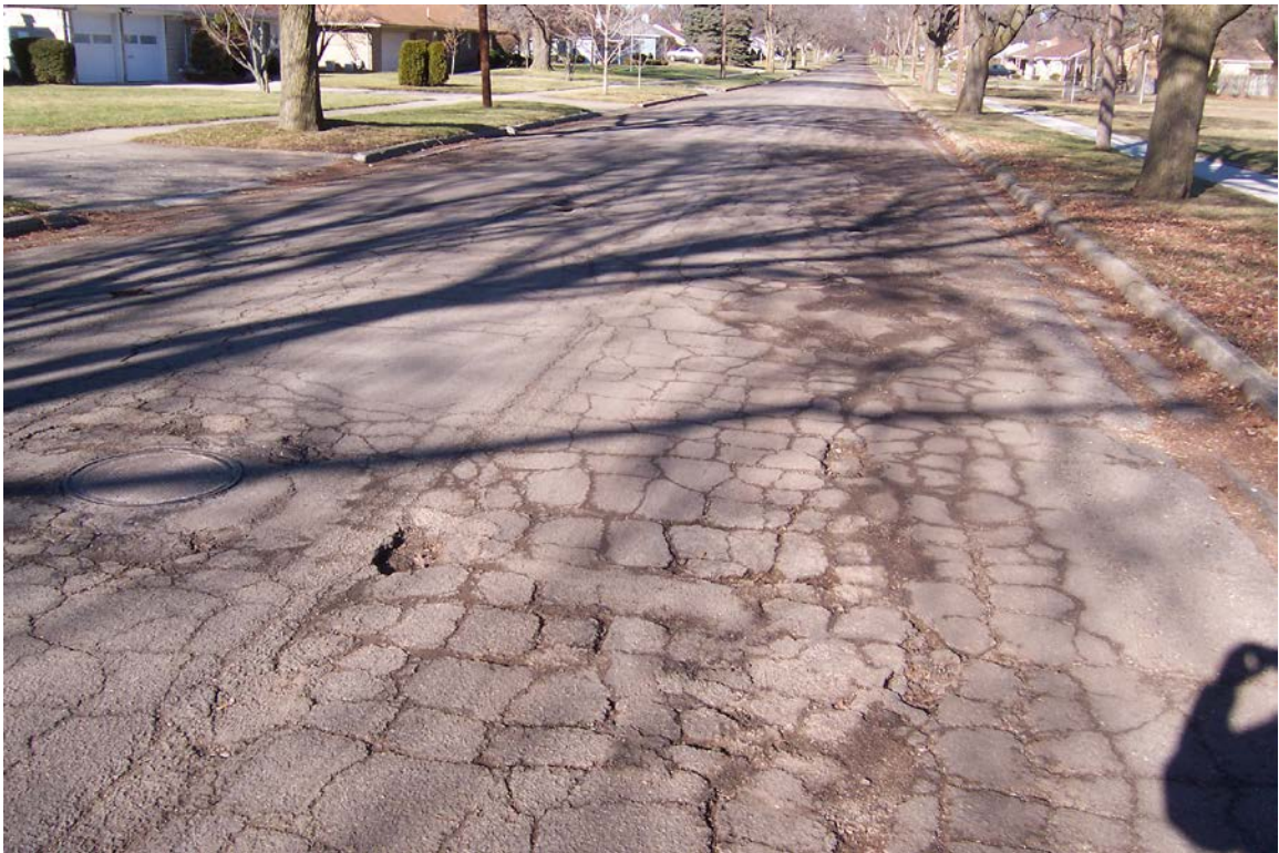
Photo 2: Facing north on Durand mid-way between south end & Oakdale ROW
