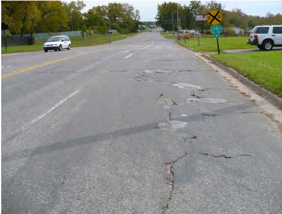
Photo 1: Facing east from south lane from east of Cooper
