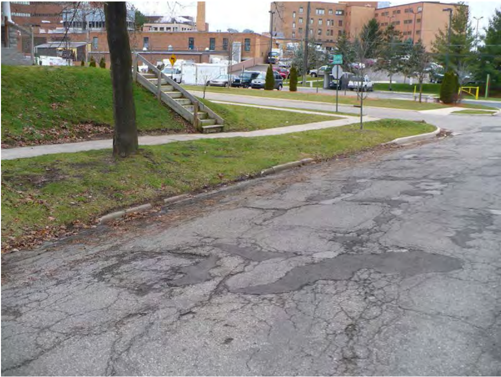
Photo 6: Condition of existing curb and gutter on south side of Homewild Avenue at Forest Avenue
