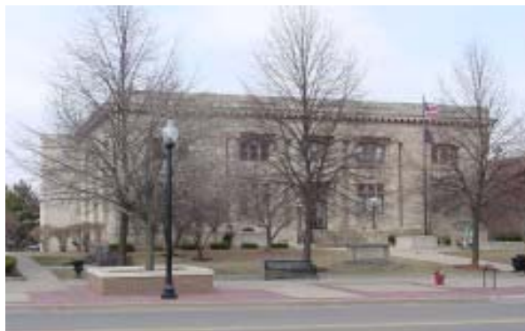
Carnegie Branch Jackson District Library
